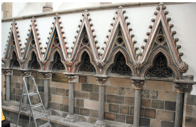
Worksop Priory former reredos - prior to restoration
