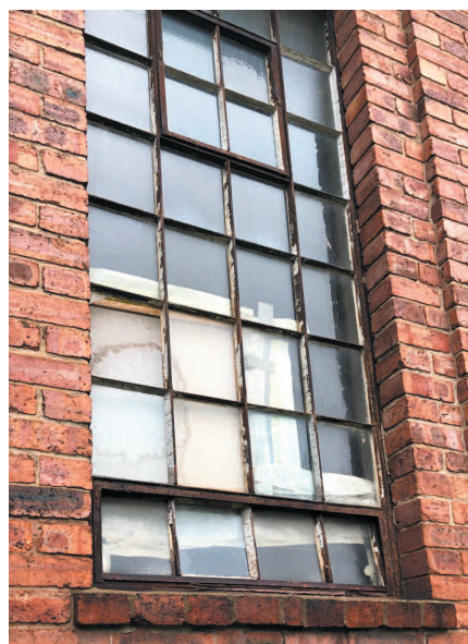
Original Crittall steel windows
