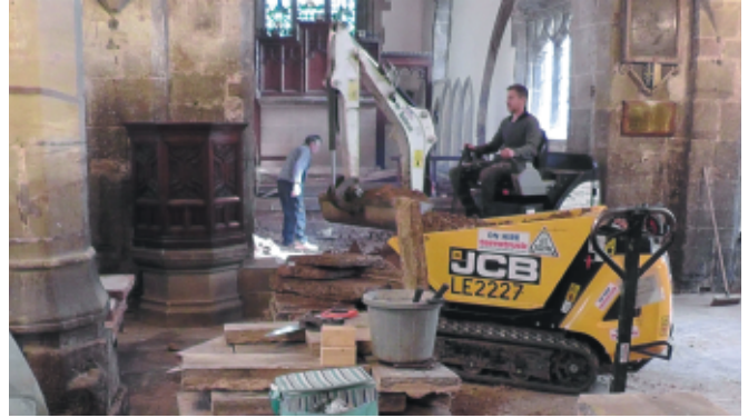
Excavation of the chancel floor
