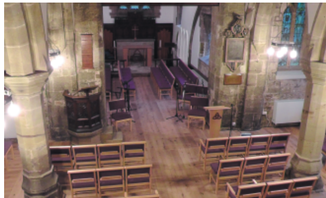
Project completed - the finished floor
