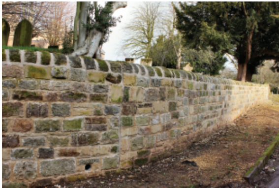
Bilsthorpe, recently repaired boundary wall.
