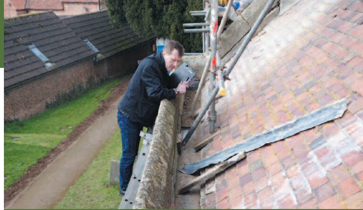
Lead replacement at St Helena's, Thoroton
